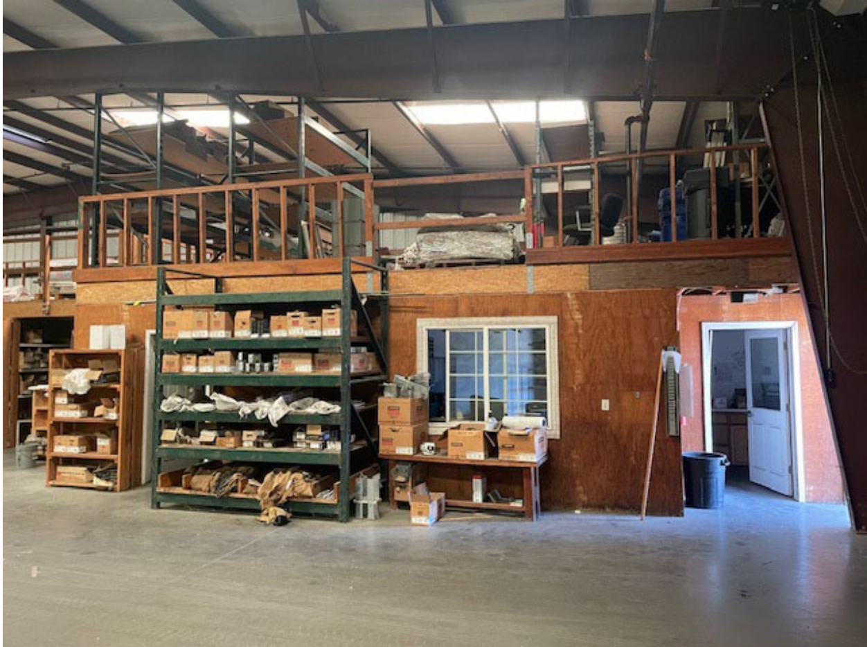
Mezzanine Inside Warehouse with Office Space and Restroom
