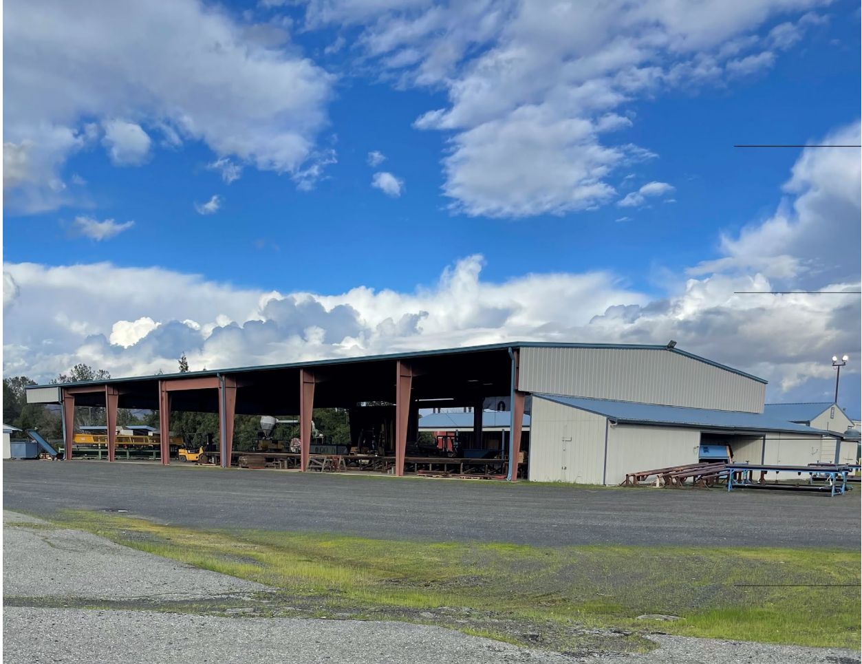
Large Equipment Covered Parking
